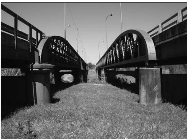
Fig. 4: The Aberdeen Bridge duplication was a successful collaboration between engineering and heritage conservation. The older wrought-iron lattice-girder bridge, shown to the left, was duplicated by a new steel Warren-truss bridge shown on the right. It was an elegant solution but one which had no precedent as a heritage conservation action within the DMR (now RTA) at the time. Richard Mackay
